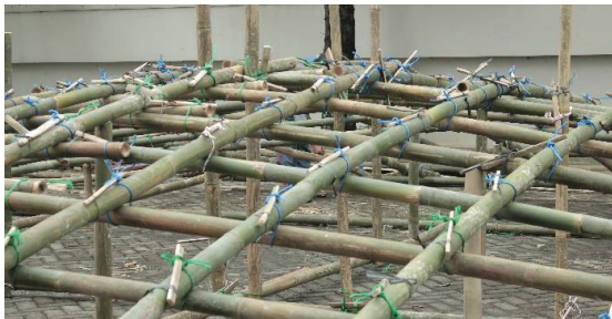
Figure 11: The connections and the temporary supports
