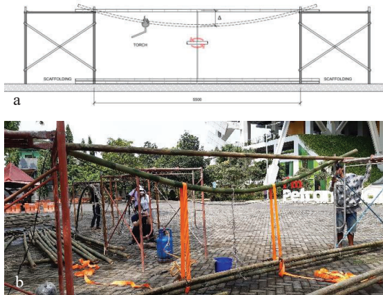
Figure 3: Setting up of bending test on the construction site
