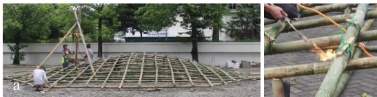
Figure 12: Heating and pulling the gridshell using chain block to add height
