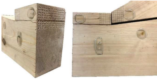
Figure 4.1: Characteristic shear failure on the tie beam-end observed in the 40 SSJ specimens tested.
