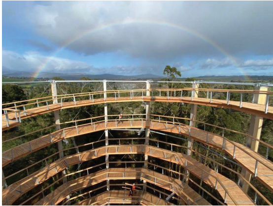
Figure 1: Viewing tower at the Avondale Forest Park in Ireland built with locally grown Douglas fir. Source: WIEHAG GmbH.
