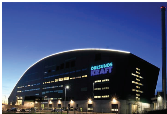
Fig. 5. Filbornaverket in Helsingborg, Sweden, is a modern waste-to-energy incineration plant that uses combustible household and commercial / industrial / demolition waste to produce 78MW of electricity and steam for district heating. It was designed to exceed EU standards for cleanliness of exhaust gases [41]. Around half of Sweden's municipal solid waste is burned for energy recovery at end-of-life, the other half is recycled [42]. Photo : Öresundskraft
