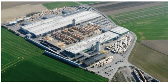
Fig. 2. Wiehag's glulam plant at Altheim near Stuttgart. Photo: Wiehag
