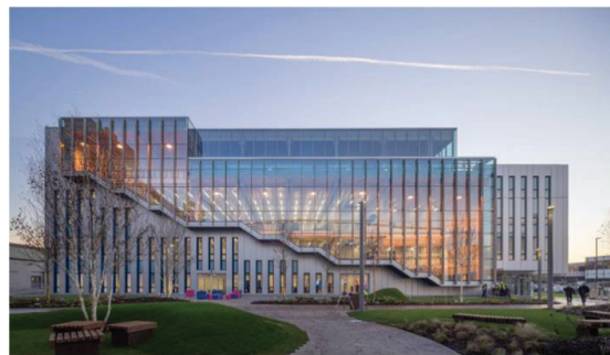
Fig. 1. The timber in this prefabricated office building for Sky UK represents -1442 t biogenic CO 2 , ie sequestered from atmosphere. Emissions from manufacture and transport from Austria represented +200 t, leaving embodied CO 2 of -1242 t (Module A1-A5 including biogenic). The alternative structure with steel frame and concrete slabs would have cost +553 t embodied CO 2 (A1-A5), ie emitted to atmosphere [44]. Given the building’s energy saving features like rooftop PV, LED lighting and CCHP, the -1242 t CO 2 represents about 13 years of operational emissions. Even if the sequestered carbon is returned to atmosphere at end-of-life, the 353 t benefit (553 t – 200 t) of the steel/concrete composite alternative, remains. Photo copyright Simon Kennedy.
