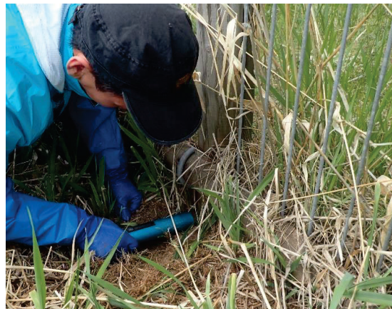
Figure 1: A scene of driving a Pilodyn pin into a pillar
