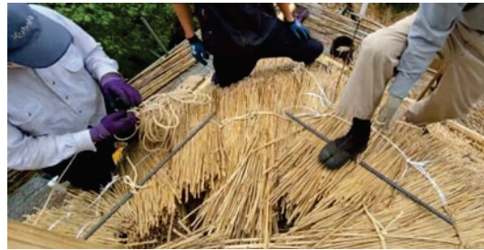
Figure 9: Reinforcing bars are used for the top shavings that support the water bottle
