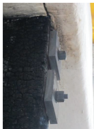
Figure 12: Tendon anchorages after test
