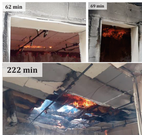
Figure 13. Test 5 failure stages of the protected TFA ceiling.
