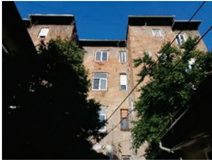
Figure 2: The eastern façade (face) of the structure
