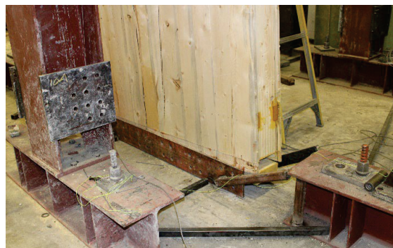
Figure 11: Specimen 1: wall withdrawal from sole plate.
