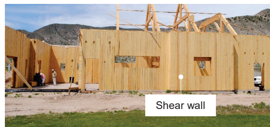
Figure 1: Interlocking cross laminated timber structure under construction.
