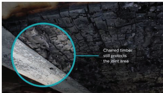
Figure 16: Specimen from below after 90-minute loaded fire test.
