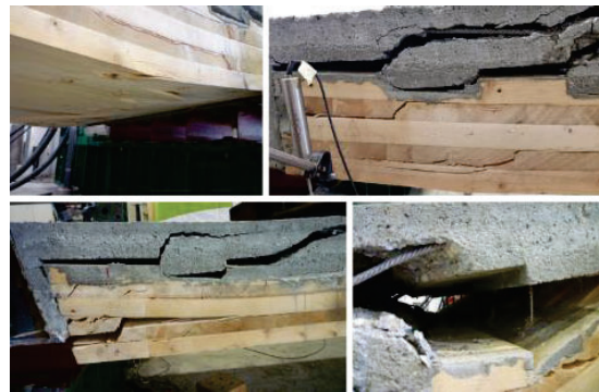
Figure 10: Failure modes in composite timber specimens: bending, rolling shear, screw pull-out and tension orthogonal to the grain (clockwise).
