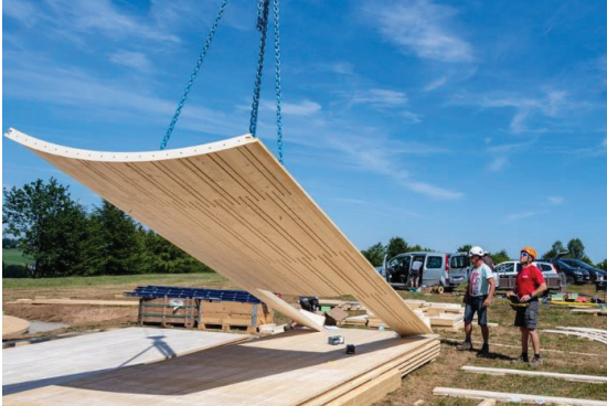
Figure 10: Lifting of curved CLT panel
