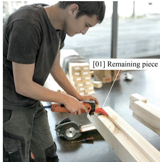
Figure 9: During assembly, the remaining piece was removed by hand with an oscillating tool.
