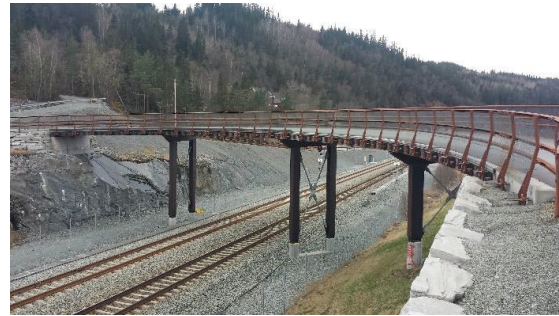
Figure 20: Plate bridge with stress-laminated deck in Hell, Norway as flyover road bridge over railway from 2009. Photo: Martin Cepelka.
