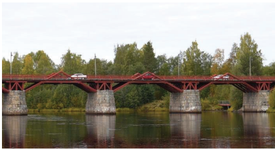
Figure 15: The Lejonström bridge built in 1737 with a combined kingpost strut-frame design is still open for road traffic. Location Skellefteå, Sweden. Photo: Per-Anders Fjellström.
