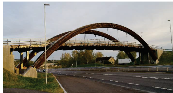
Figure 1: Vinsnes Bridge over Rv. 22 near Lillestrøm in Norway from 2015. Design: COWI AS. Photo: Martin Cepelka.
