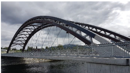
Figure 22: Network arch bridge with concrete deck and timber arches. Steibrua in Alvdal, Norway from 2016. Photo: Martin Cepelka.
