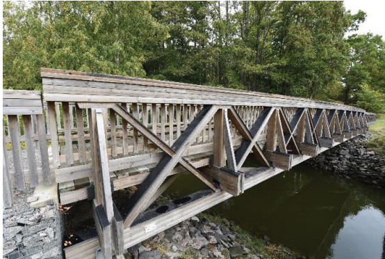
Figure 27: Pedestrian Howe Truss bridge to Källandsö close to Lidköping, Sweden. The design is a 25m truss bridge with a transverse plank deck. Built 2017 by Martinsons. Photo: Per-Anders Fjellström.
