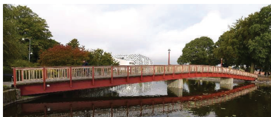
Figure 26: Pedestrian bridge to Strömsholmen in Eskilstuna, Sweden. The design is a 48 m 3-span beam bridge with a transverse plank deck. Built 2001 by Svenska Träbroar. Photo: Per-Anders Fjellström.
