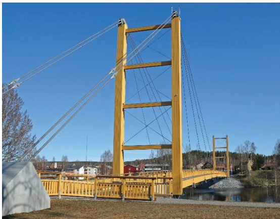
Figure 28: Älvsbackabron is a cable-stay pedestrian bridge with a 129m span built 2012 over Skellefteälven, Sweden, by Martinsons. Photo: Per-Anders Fjellström.
