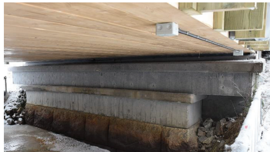
Figure 31: Factory installed M.C-sensors in a stress-laminated deck provide the owner with reliable data from inspections. Road bridge built 2022 by TBS, Junsele Sweden. Photo: Per-Anders Fjellström.
