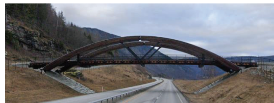
Figure 21: Arch bridge as flyover road bridge over E6 near Sorperoa, Norway from 2016. Photo: Google.
