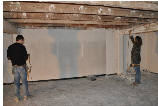
Figure 4. Beam inspection with acoustic waves in the building
