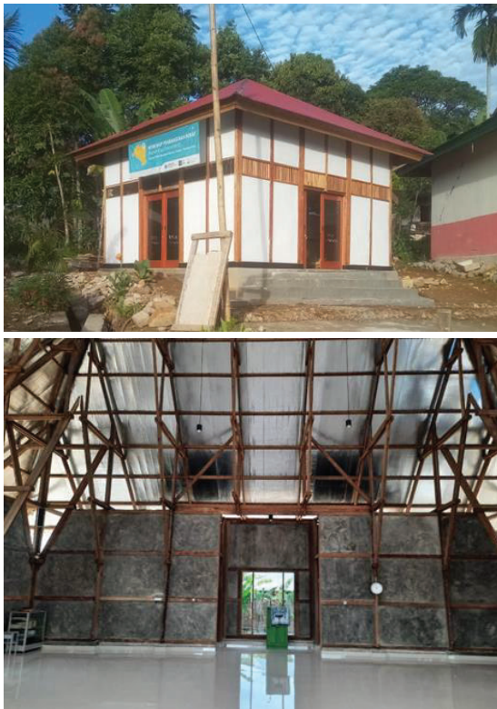
Figure 30: Musholla in Pasaman (left) and Al Munawarrah mosque in Mamuju (right) using ferrocement wood wall construction.
