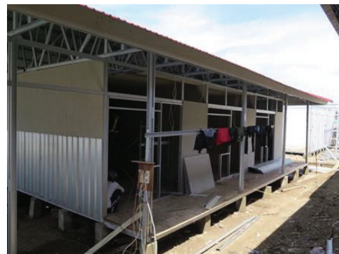
Figure 1: Shelters built in Petobo, Palu, using light steel, spandex roofs and GRC walls.
