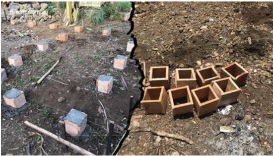
Figure 7: Local foundation construction at a house site in Mamuju.
