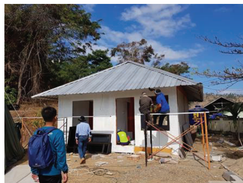
Figure 2: Model house using risha concrete frame and GRC wall covering.
