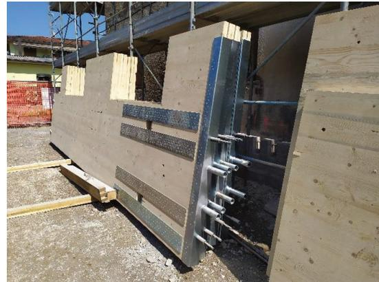
**Figure 6:** Prefabricated CLT panels ready to be installed
