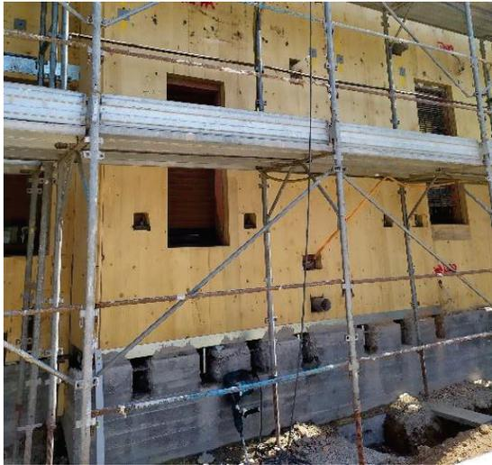
**Figure 8:** Panels arranged on the façade and connected with the new foundation
