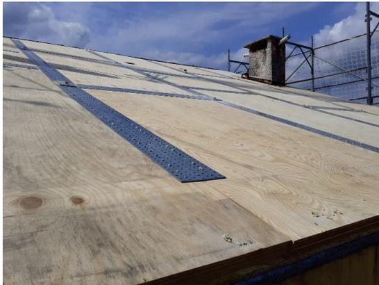
**Figure 9:** Construction of the diaphragm at the extrados of the existing roof
