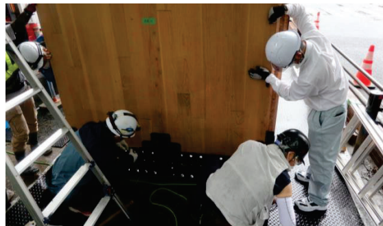
(d) Jointing the walls and the steel base with bolts
