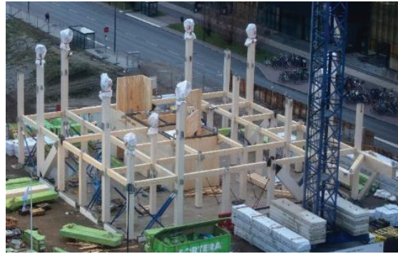
Figure 15: On site situation the 6th of December 2022. Picture taken from south-east.
