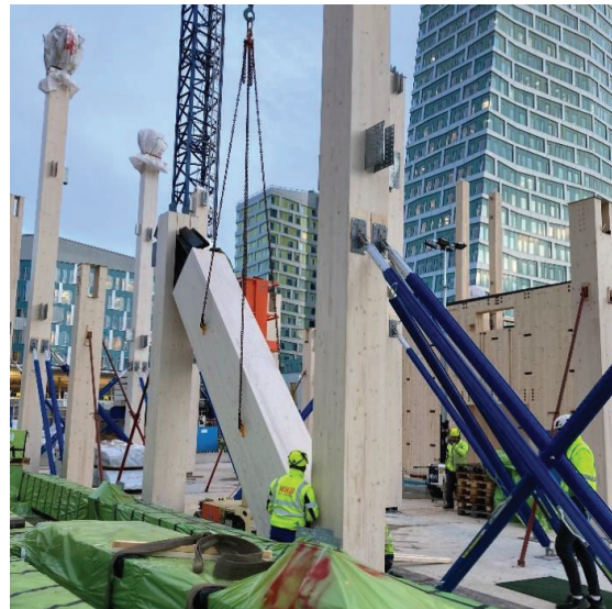
Figure 7: Bracing beam during installation
