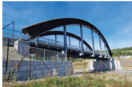
Figure 15: Tande Bridge open and in use. Picture taken by Sweco
