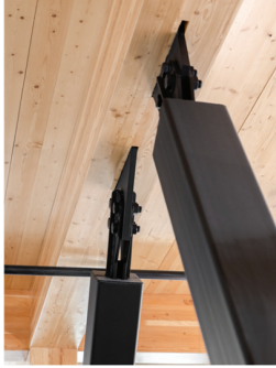
Figure 4: Painted Brace Apex Connection
