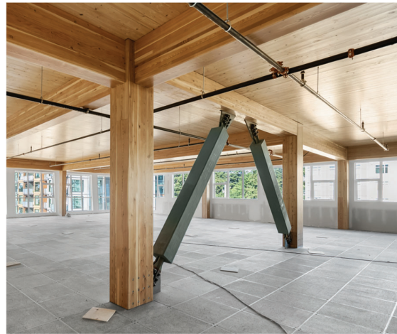
Figure 3: Newly Installed Braces
