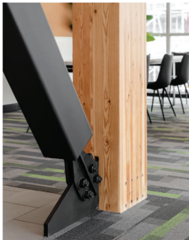
Figure 5: Painted Brace-Column Connection
