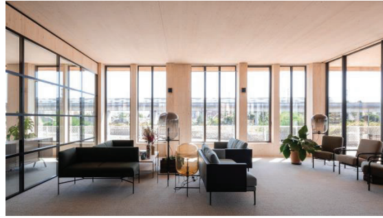
Figure 3: Mock-up of the office floor, with visible CLT ceiling © WO 2
