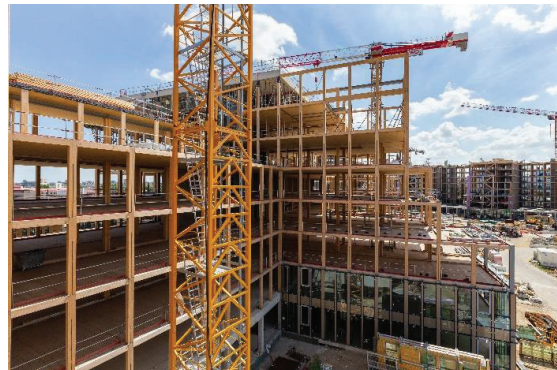
Figure 4: View of the construction site (Aug. 2022) – © Raffin
