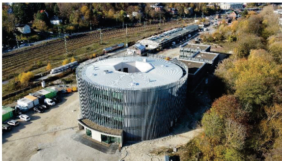
Figure 5: Aerial photo with main building in foreground
