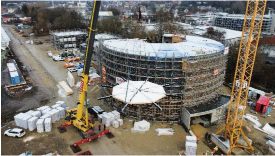
Figure 8:: Lifting of the subtensioned system
