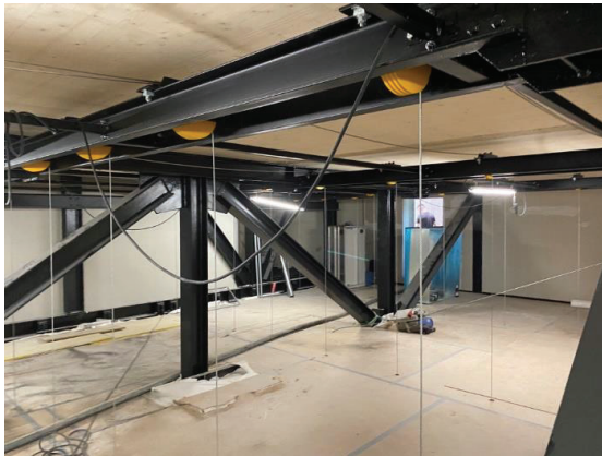
Figure 16: Trusses in the area of the lacing floor
