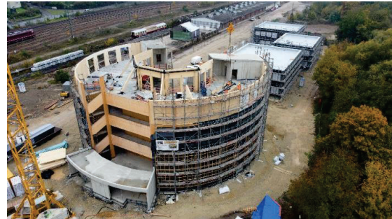
Figure 6: State of construction of the main building
