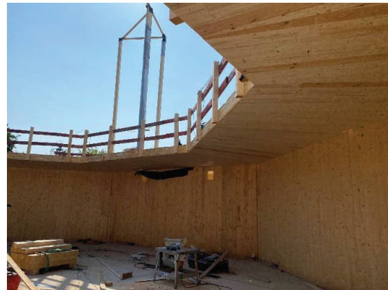
Figure 13: Cantilevered ceiling elements in the as-built condition
