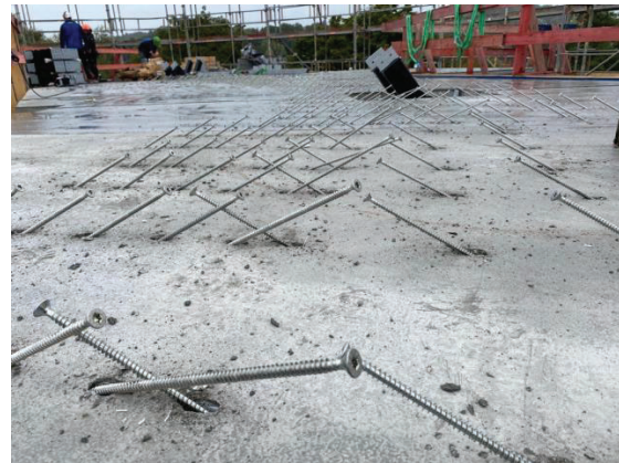
Figure 14: Screwing the concrete slab at the construction site
