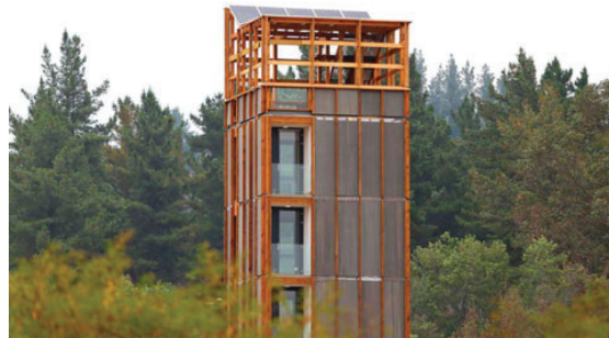
Figure 7: Experimental Tower with 6 floors. Peñuelas, Chile.
