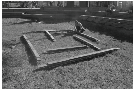
Figure 6: Preassembled units for a novel slide-in connected, planar reciprocal frame structure. The units are assembled from salvaged wood by the use of wooden nails.
