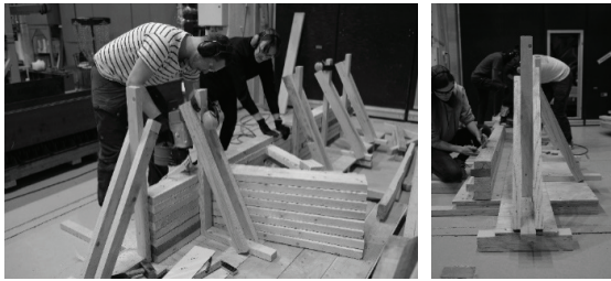
Figure 4: Working process using templates and guides for precise fabrication of bespoke plaza elements
