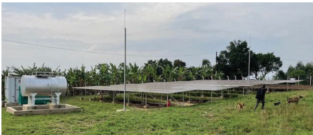
Fig. 15. The Katarwe village 56-kWp solar mini-grid was installed by NRECA in 2022 for USAID Power Africa and operated by the local KRECS utility. This system provides 3-phase power to 176 households, several small stores, two dairies, a coffee factory, and a telcom mast. (Credit: Robert Foster)
