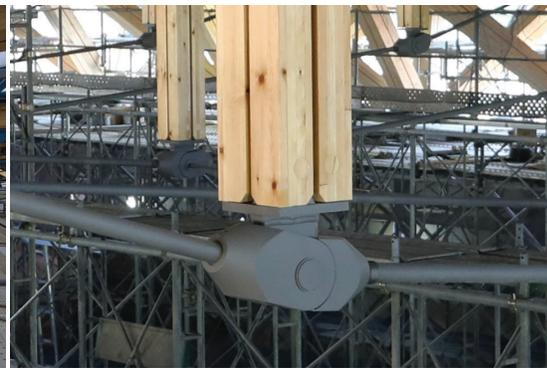
Figure 22. Connection between the string and the strut
