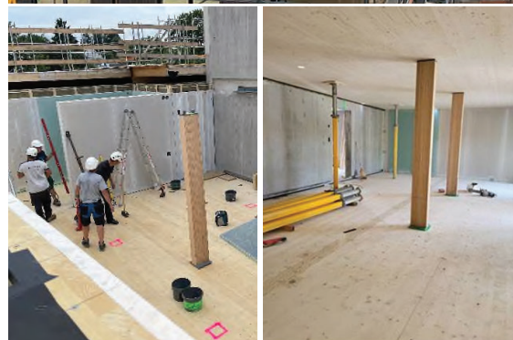
Figure 12. Construction site of “Im Zelg” in Uster: Floor-panel layout (top), preparation of bearing support and inside view under construction (bottom), Source: Timber Structures 3.0 AG
