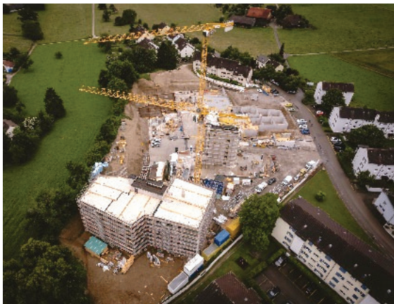
Figure 10. Top view on the construction site of “Im Zelg” in Uster. The first building is being erected, the concrete core of the second building is being built and the basement for building 3 is being constructed. Source: Timber Structures 3.0 AG
