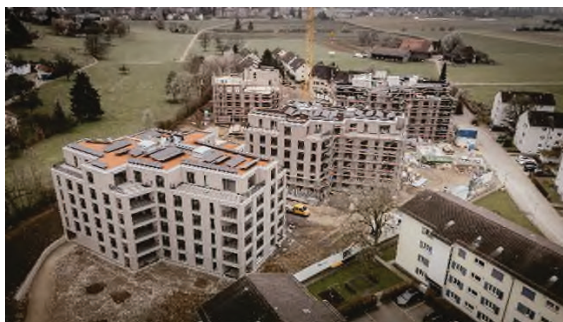
Figure 11. View of the construction site at the beginning of 2025, with the first building erected and buildings 2 to 4 in various stages of construction in the background. Source: Timber Structures 3.0 AG
