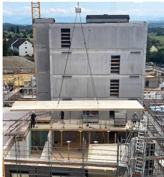
Figure 10. Top view on the construction site of “Im Zelg” in Uster. The first building is being erected, the concrete core of the second building is being built and the basement for building 3 is being constructed. Source: Timber Structures 3.0 AG
