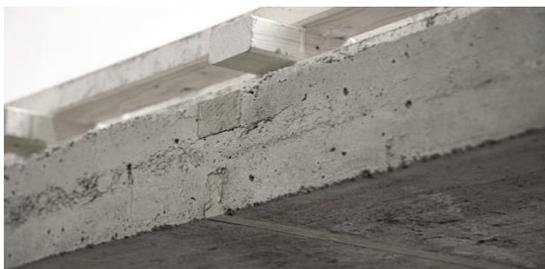
Figure 2: Prototype of a timber earth slab [1]
