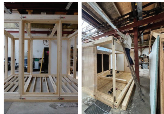
Figure 116. Basic load carrying structure formed by L-shaped profiles to receive layers (left) and experimentation on gable wall.
