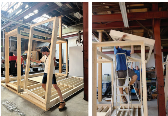
Figure 10. Assembly of the elements that can be carried out by two un-skilled workers at most, not exceeding 25kg per worker. No special equipment is necessary.
