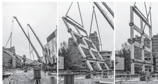
Figure 8. Example of Pres-Lam tilt-up construction
