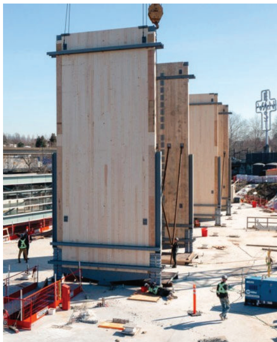
Figure 5 – Shear wall construction in The Hive project. Photo by Ventana Construction Corporation (Matthew Marsolais).
