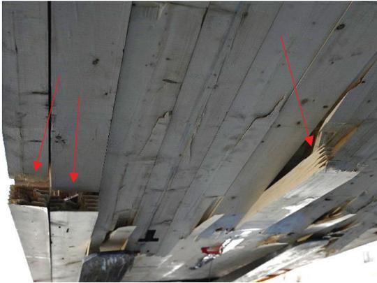
Figure 6: Prominence of finger joint failure
