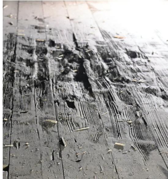
Figure 8: Charring and warping of fibres
