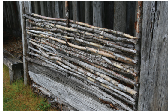
Figure 3: Timber fences that utilize the natural shapes of tree branches and twigs through interlocking in the Viking village near Vestrahorn, Iceland.
