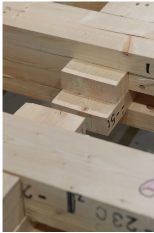
Figure 15: Slide-in connection that allows over-length of timber boards.
