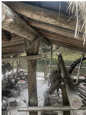
Figure 6: An example of using tree forks to support a beam in Jiangxi Province, China.
