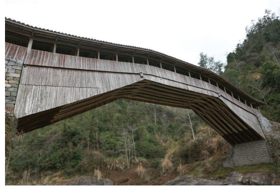
Figure 7: Xianju Bridge: a typical woven timber arch bridge in southeast China.
