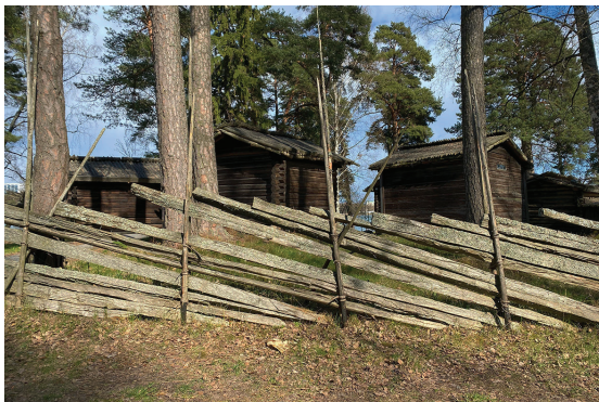
Figure 1: Niemelä tenant farm: timber fences using small tree branches and split timber; Seurasaari Open Air Museum, Helsinki, Finland.
