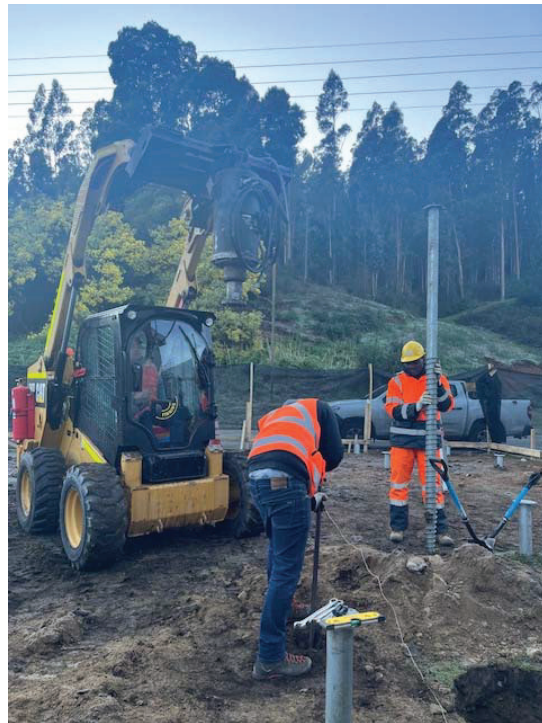
Figure 8. Installing foundation screws with an auger drill at a construction site
