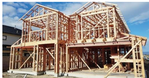
Figure 1. A typical LTF building under construction
