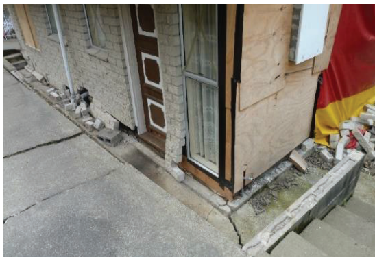
c) A red-sticked down-slope house with temporary cladding
