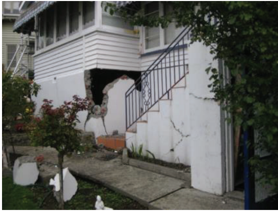
a) Significant damage to brick foundation walls
