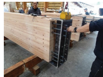
(b) Setting steel connection at beam end
