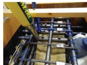
(c) Mortar injection at mechanical joint in the centre of rebar
