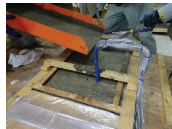
(d) Casting concrete at column and beam intersection
