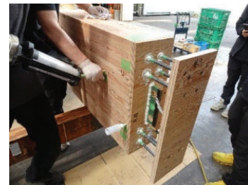
(a) Glue injection at beam end
