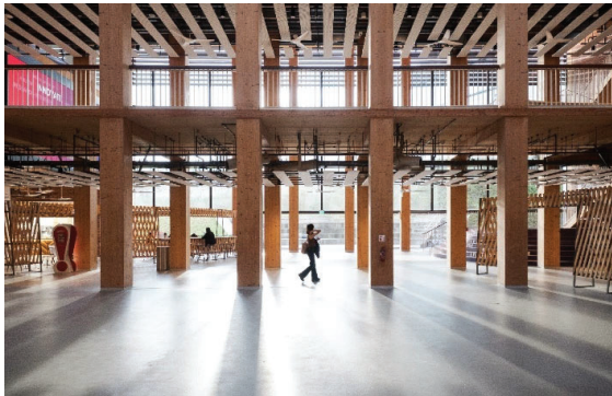
Figure 8 - Gaia exposed internal MET structure and finishes (source NTU Singapore)
