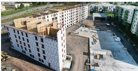
Figure 3. Light wood frame structure Project: Le Prisme Logisco, Photo credit: Le natif
