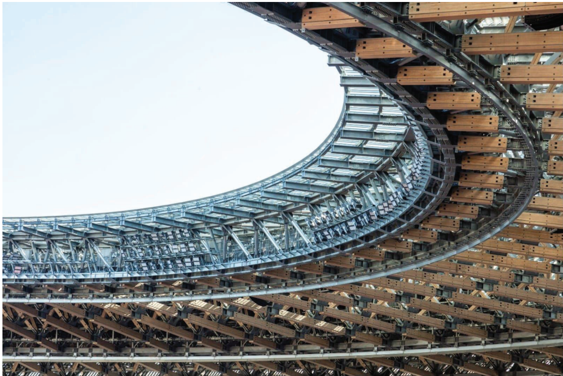
Figure 4. Japan National Stadium in Tokyo utilising timber beam as part of the roof structure © Kengo Kuma Associates
