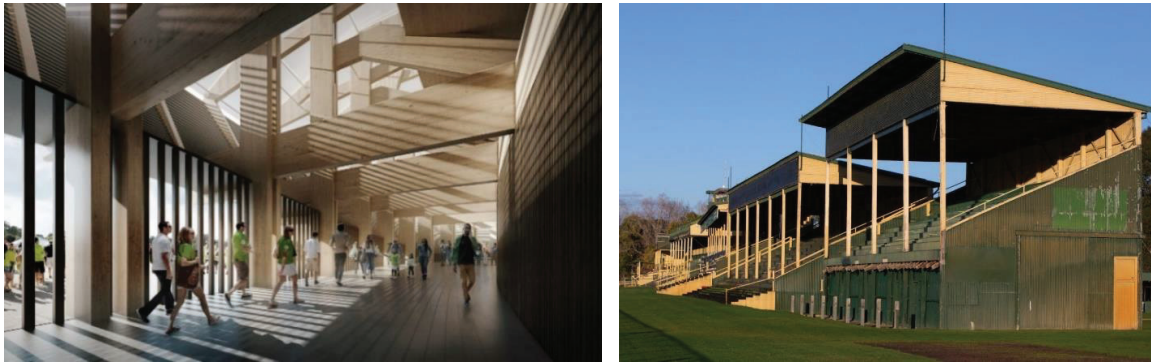
Figure 1. Mass Timber Framed Stadia Concept © Zaha Hadid Architects (left) vs Lightweight timber frame grandstand © Brett Hartwig/InDaily (right)
