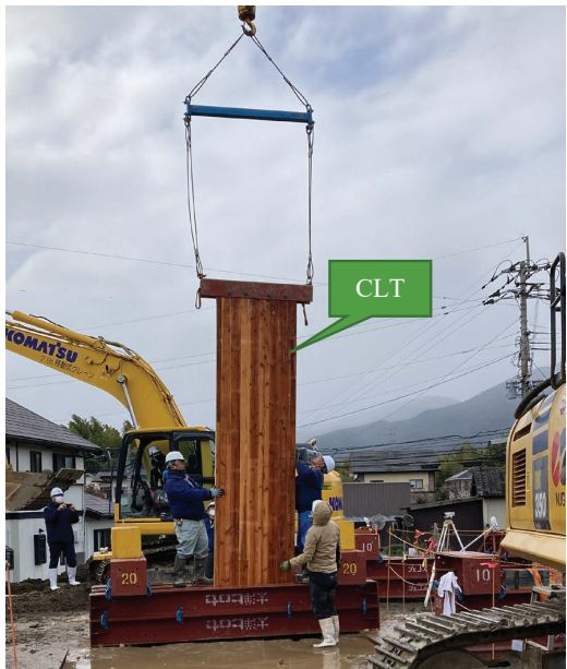
Figure 7. Inserting CLT into the ground
