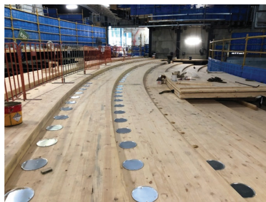
Figure 9. Lower stalls with covers over seat post diffuser penetrations (Courtesy: Arup)
