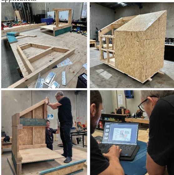
Figure 13. Small-scale mock-up prototypes constructed at Fairweather Homes' factory
