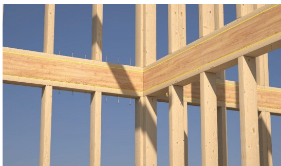
Figure 1. Example of typical structural joints with interposed acoustic layer (Rothoblaas archive).
