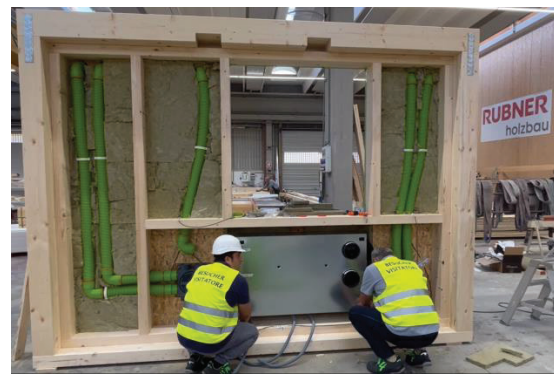
Figure 9. Mock-up realization, VMU and ventilation ducts integration
