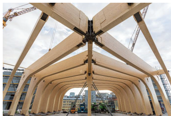
Figure 13 Cover plates around star node
