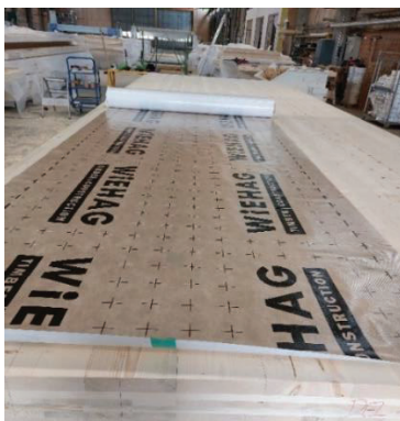
Figure 26 timber protection on all floor areas
