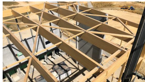
Figure 15 bracing of the roof
