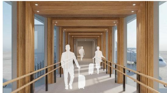
Figure 3: CLT wall columns and roof structure (interior perspective)
