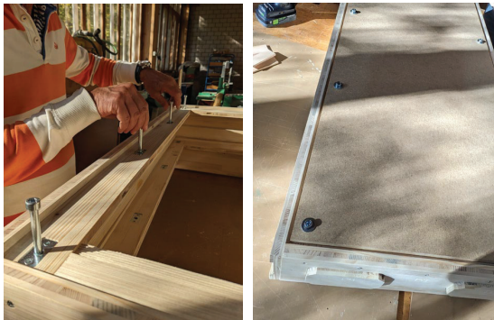
Figure 9. Matching holes between the wall and the layer in a mock-up wall.
