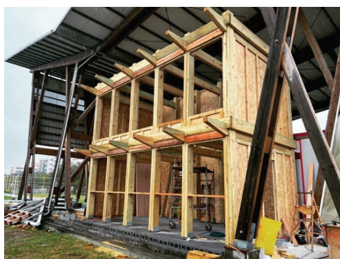
Figure 7 Demo House built in DLT
