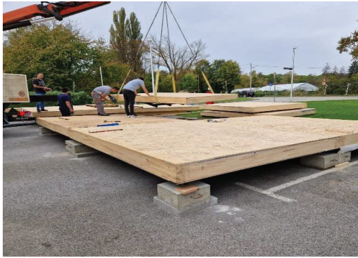
Figure 8 Preparation of floor assembly
