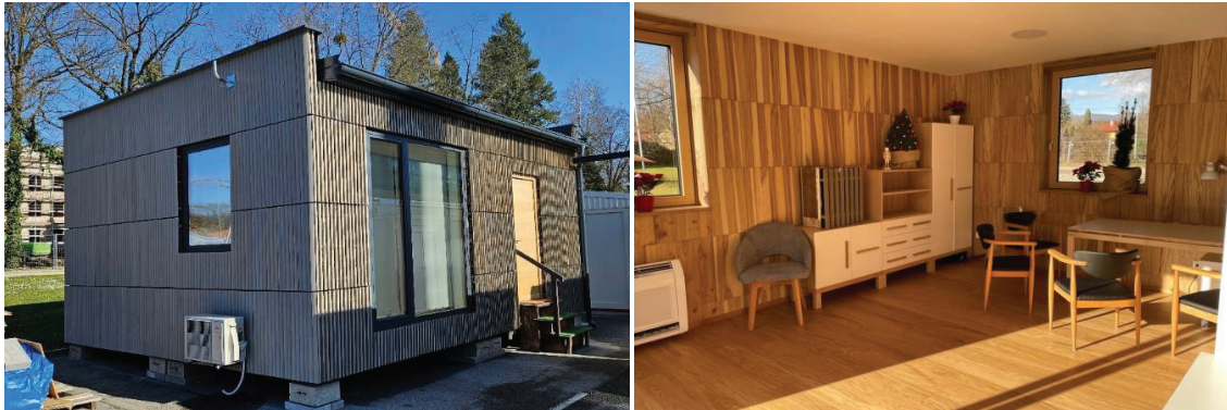
Figure 4 View of the finished experimental bungalow from outside showing ventilated oak wood cladding (left), interior view demonstrating different appearance classes of panelling (right)
