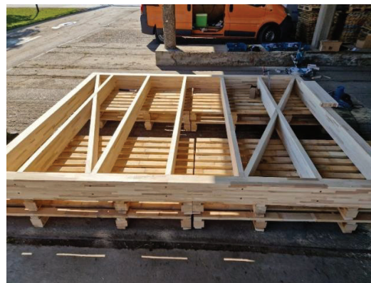
Figure 7 Preparation of load bearing walls
